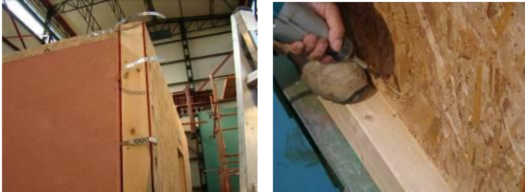
Figure. 3: Connection of walls with screws.
